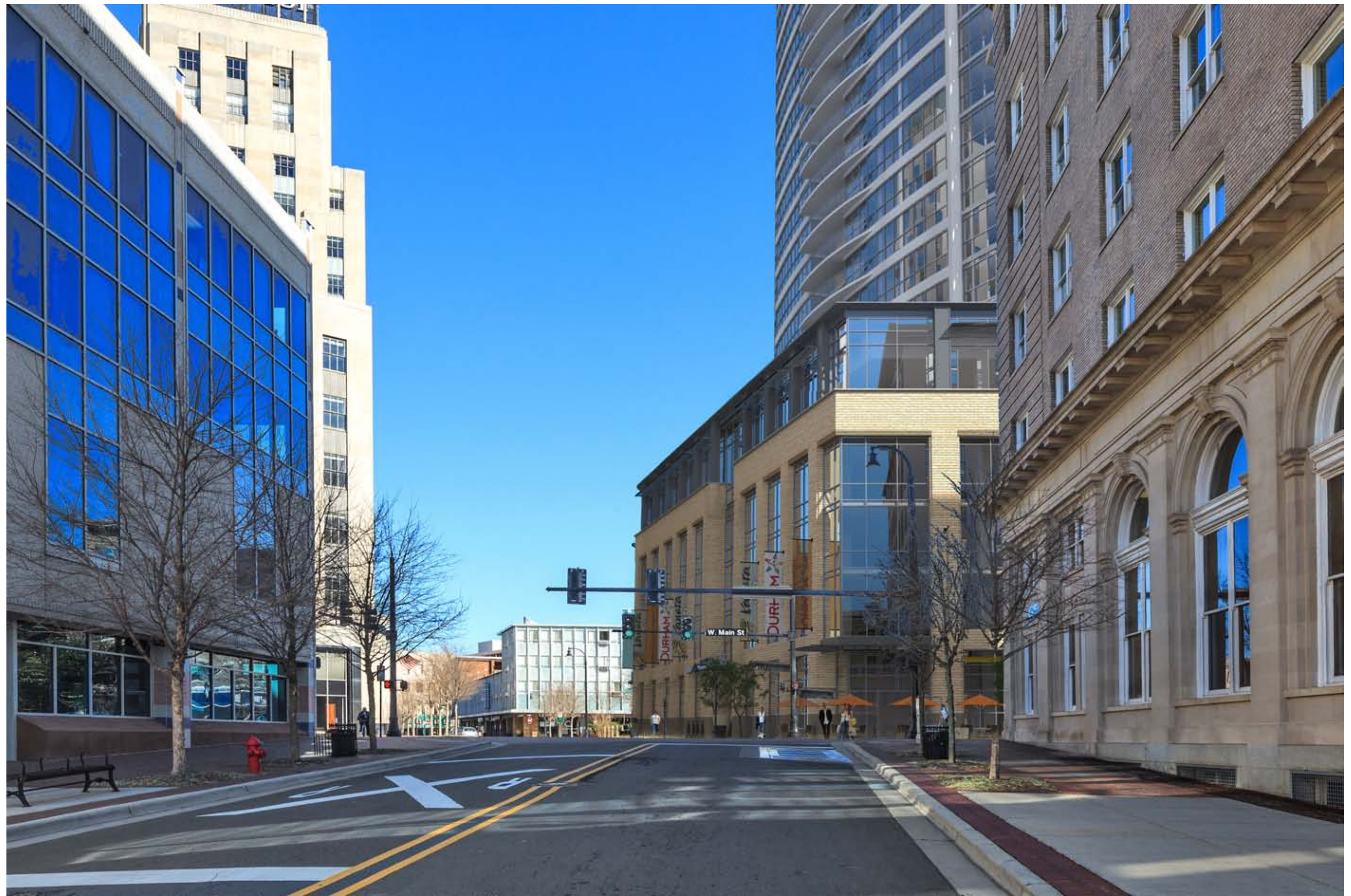
Close-Up Perspectives: North Corcoran Street View From South Of Site
